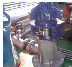
Compact installation of a seepex BE range pump directly on the tank
