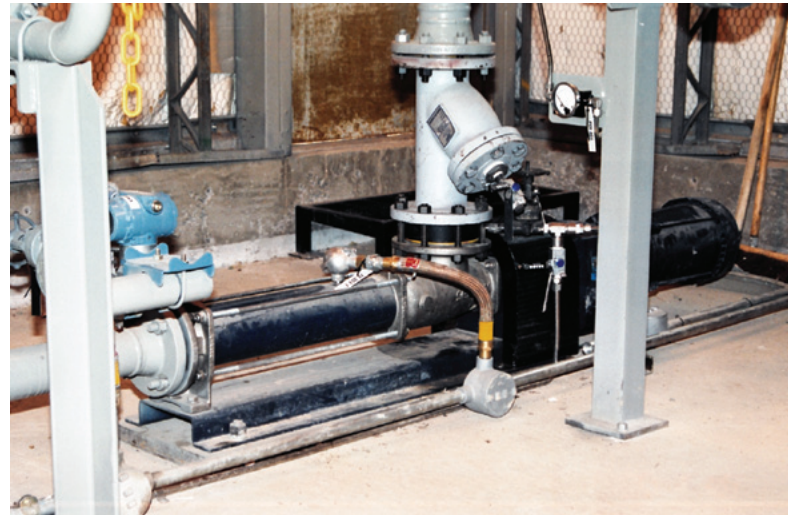
seepex progressive cavity pumps offer a wide range of cost effective pumping solutions for boosting and transfer of oil, gas and produced water
