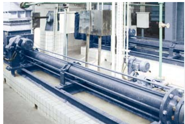
Pumps of range BTI 35-48 Conveying product: Dewatered sludge Conveying capacity: 16 m 3 /h (70 GPM) • Pressure: 35 bar (507 PSI) Temperature: 20 °C (68 °F)
