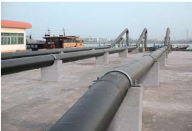
Long distances seepex pumps convey dewatered sludge over long distances – even over 200 m (650 ft).
