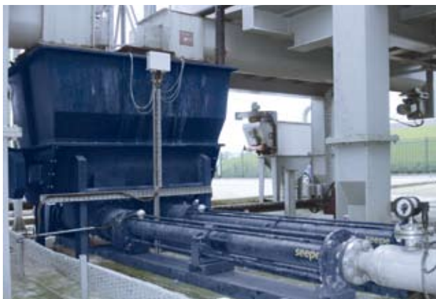
Pumps of range BTEI 17-48 with 6 t buffer hopper with live bottom Conveying product: Dewatered sludge with a ds content of 16 – 18 % Conveying capacity: 4 m 3 /h (17 GPM) • Pressure: 24 bar (348 PSI) Temperature: 20 °C (68 °F)
