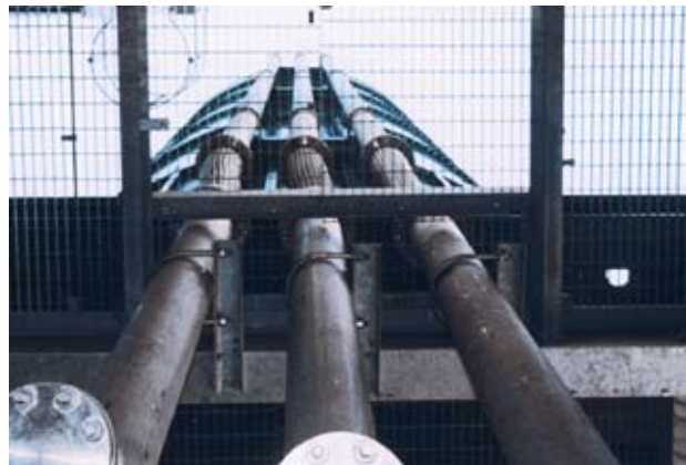
Long distances – even vertically seepex pumps not only convey dewatered sludge horizontally over long distances. Vertical head – 30 m (98 ft) to silo top – is not a limitation.
